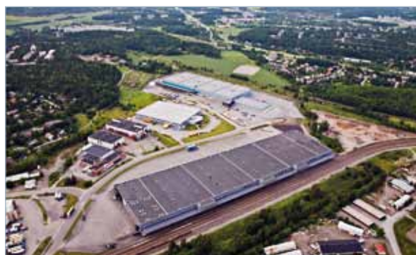
Posten Logistik SCM Oy's logistics centre's topping out party in August
