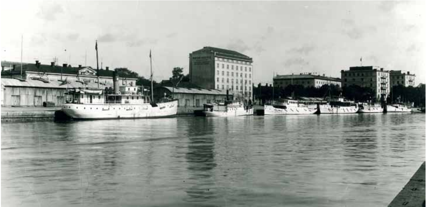
Lower steamship harbour in 1939. The construction of Martinsilta Bridge started during the same year, and it was built where the second ship is in the picture. Later on the bridge limited the ship traffic to the quays below it. Behind the ship in the foreground you can see the old Weigh Station and the upper part of the customs warehouse. On the right Höyrylaiva Oy Bore's office and residential building which was completed in 1929.
